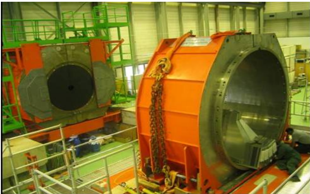
Figure CP 11: Assembled HF modules in building 186 at CERN.
