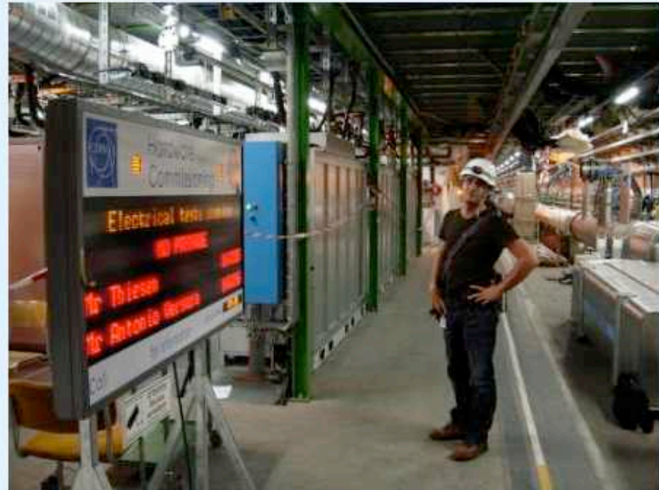
Power tests in one of the tunnel enlargements
